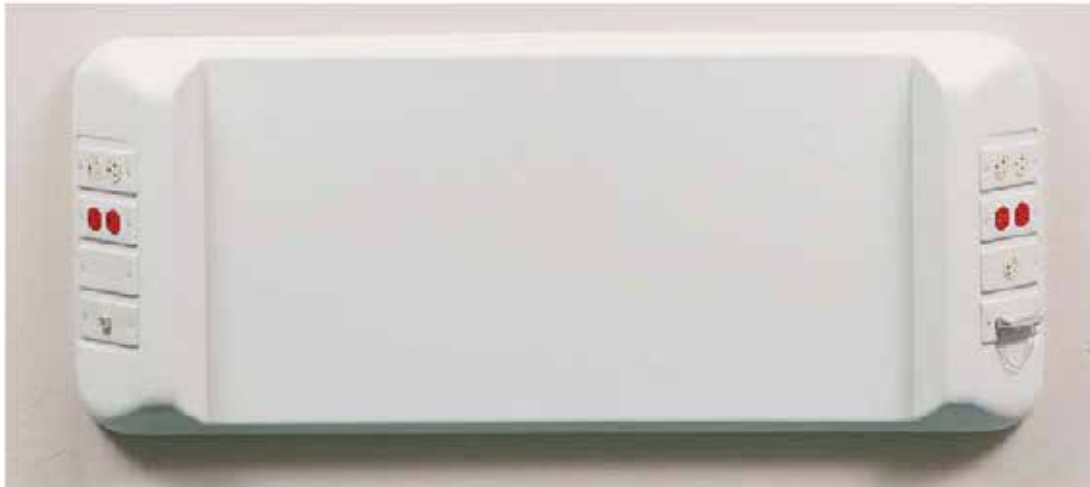
View of installed Bed Docker
